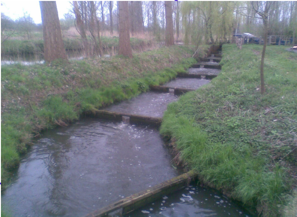
Image 5: 'Vertical -Slot' fish passage at the Hoodonk watermill, from Wouters, F., 'Visual & hydraulic research of fish passages for the De Dommel Water Board', 2012.
